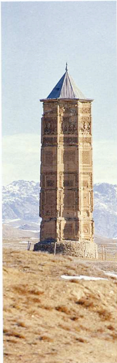
Medieval masons evolved sophisticated methods of laying bricks in patterns. Contrasting light and shadow, these designs sometimes spelled out words and phrases. The minaret built around 1100 by the Ghaznavid sultan Masud III in Ghazna, Afghanistan, is the first surviving example of this script.
