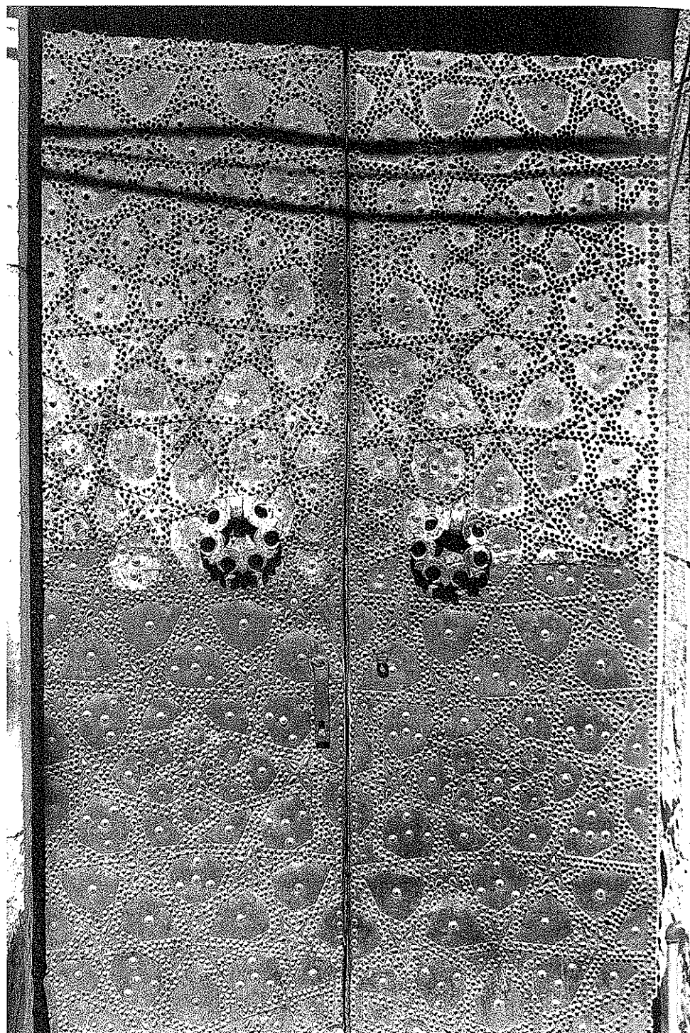
38 Damascus, bimāristān al-Nūrī, 1154. Wooden door sheathed in copper and ornamented with brass nails.
