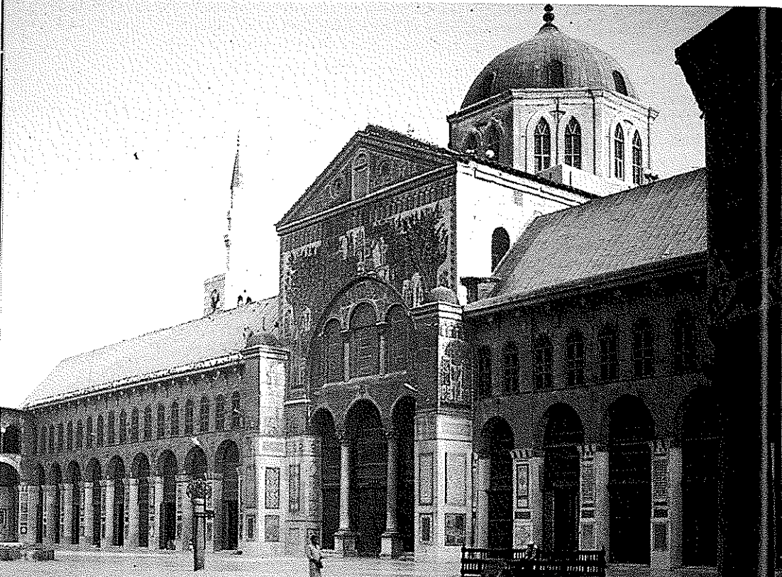
12 Christian architecture Islamicized. Great Mosque of Damascus, completed in 715 by the caliph al-Walid I. In the foreground, the treasury. The sanctuary façade and dome were rebuilt after the catastrophic fire of 1893; the original arcade would have been much lighter.
