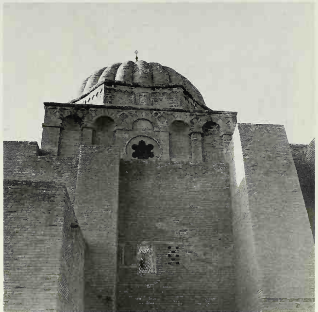
31. Qayrawan, Great Mosque, 836, 862, and 875, dome (exterior)
