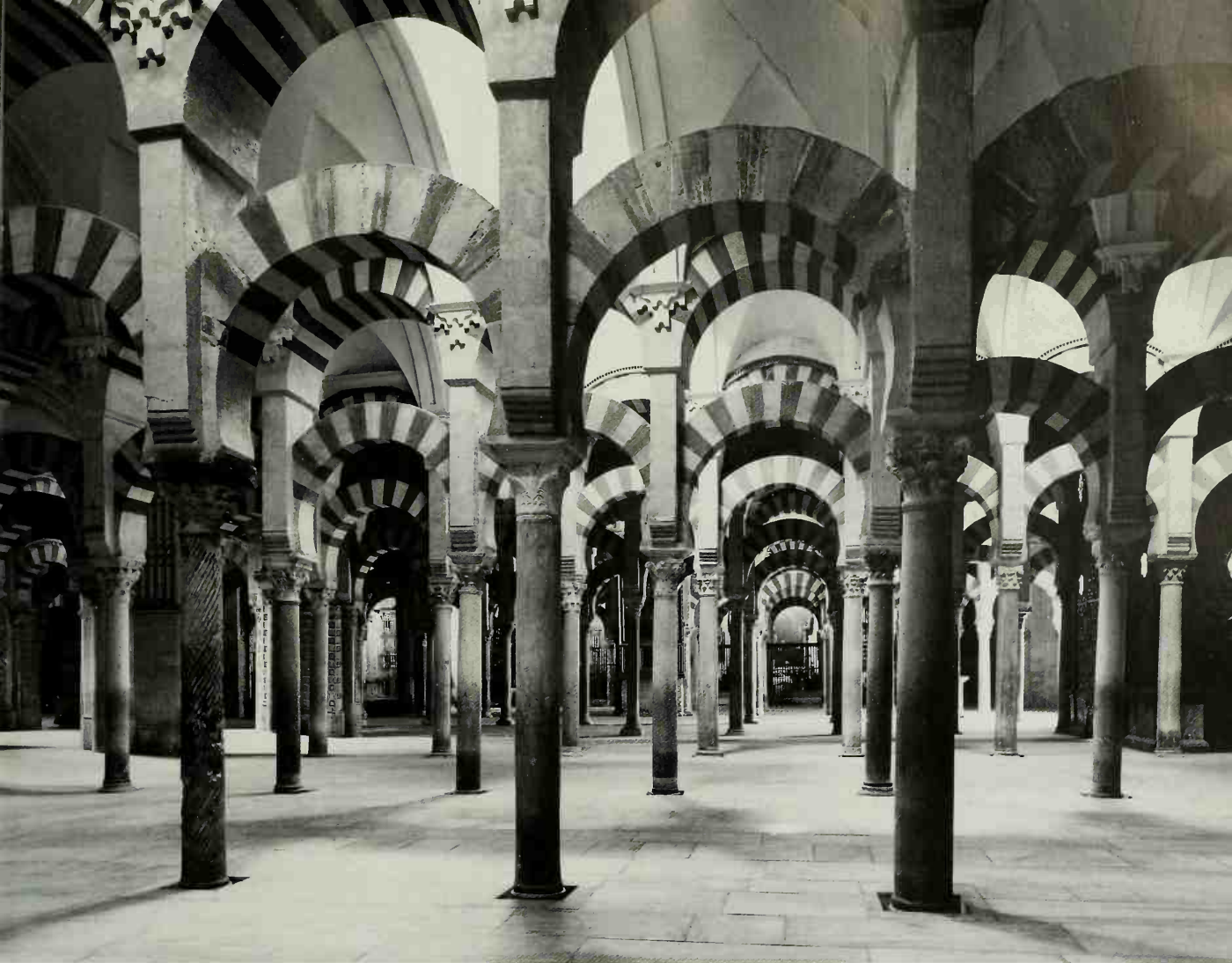
127. Cordoba, Great Mosque, al-Mansur's addition
