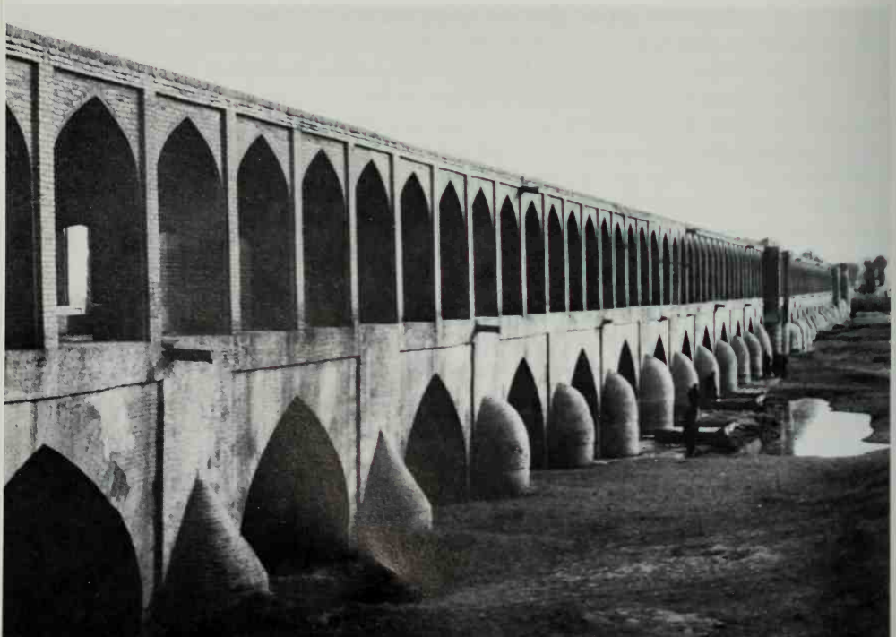
181 A Sasanian tradition revived. The Allahvardi Khan bridge, Isfahan, stretches 300 m (984 ft). Designed to carry traffic and regulate flooding with its massive buttresses; it also has pleasure pavilions.
