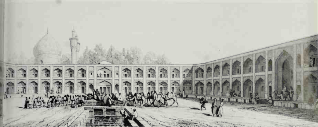
180 The hub of commerce. Caravansaray built by Shah Sultan Husa'ín with adjoining madrasa and bazaar: Isfahan, 1706–15. Spacious and austere practical, it could accommodate hundreds of animals and their loads, while the two-storied arcades held living chambers.
