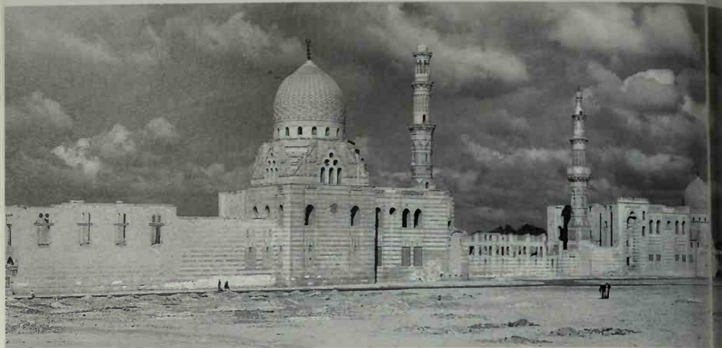
116 In the shadow of the pyramids. The Egyptian obsession with death resurfaces in new guise under the Mamluks. The funerary complex (mosque, mausoleum, madrasa , khanqah ) of Sultan Inal, 1451–6, in the so-called City of the Dead in Cairo, flouts the Prophet's insistence on modest burial.
