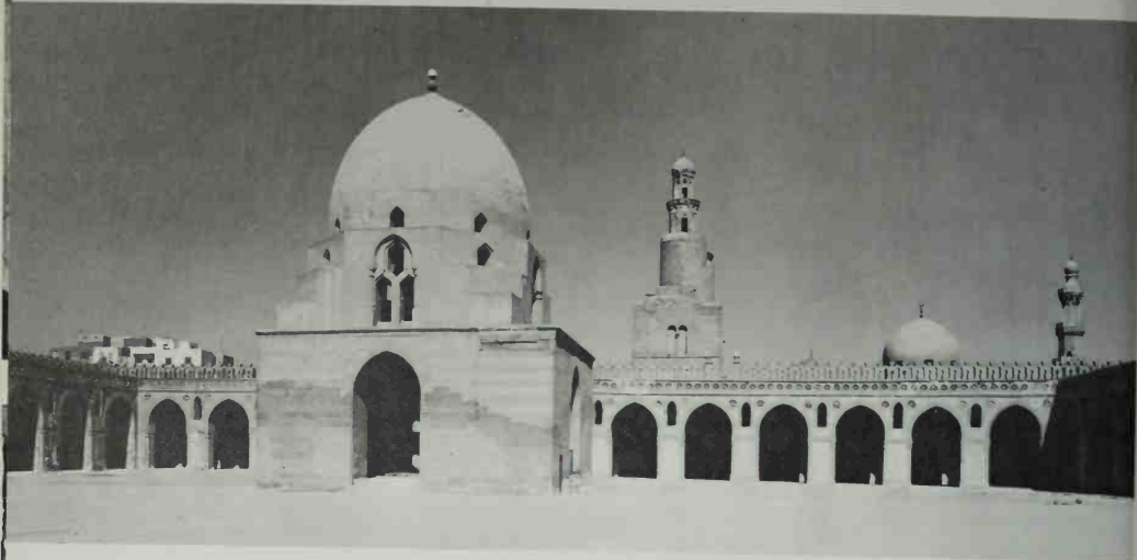
28 Courtyard of mosque of Ibn Tulun, Cairo, 876–9 (the foreground dome dates from 1296). Its essence is Iraqi: outer enclosure, brick construction, piers with engaged columns, crenellations, stucco ornament and minaret. The pointed arch serves as a leitmotif. The mosque was connected by a broad road to its patron's palace.
