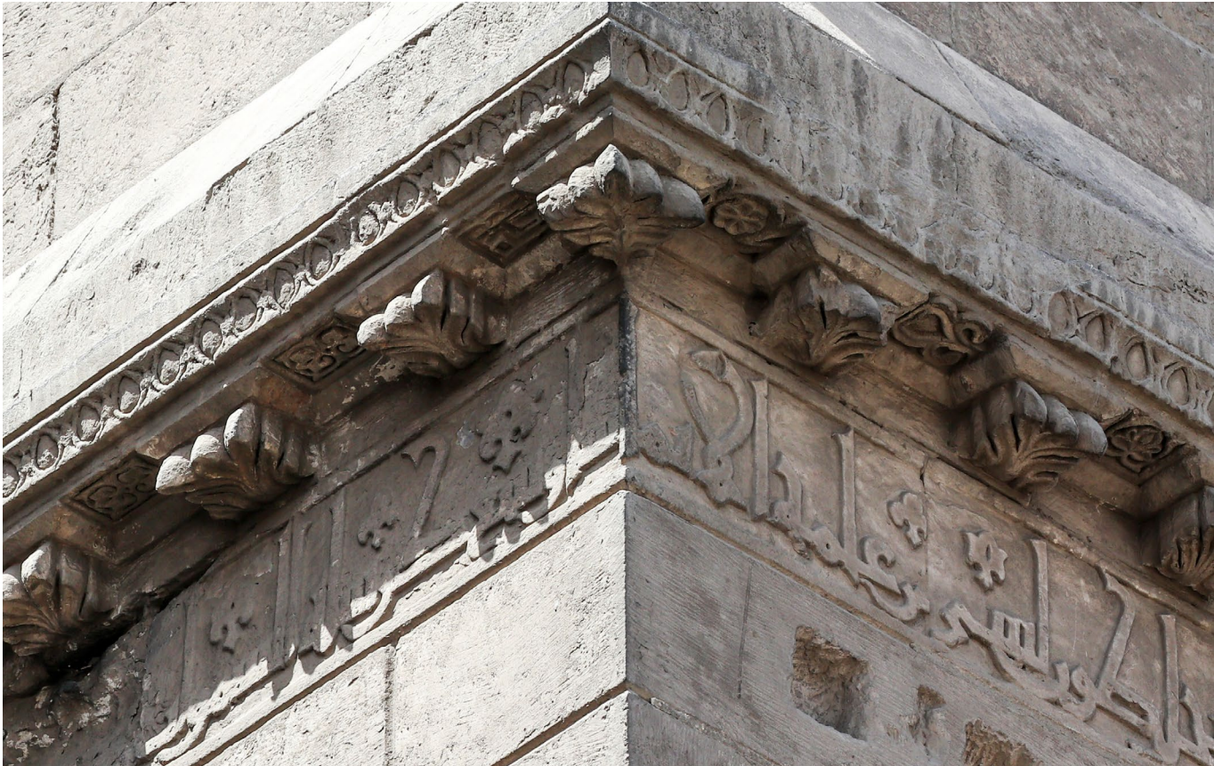
Detail of the foundation inscription of Bab al-Nasr (1087).
